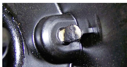
Inspect not only the distributor cap's internal contacts for burns and pits, but also ensure that the centre spring-loaded carbon unit makes contact with the rotor arm.
